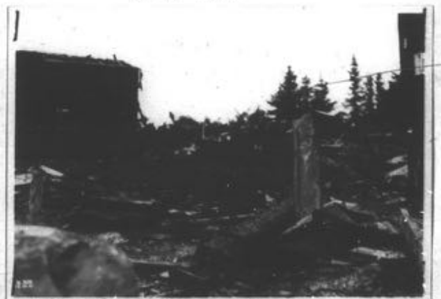
Construction Shack Fire
