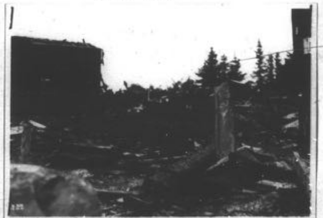
Construction Shack Fire
